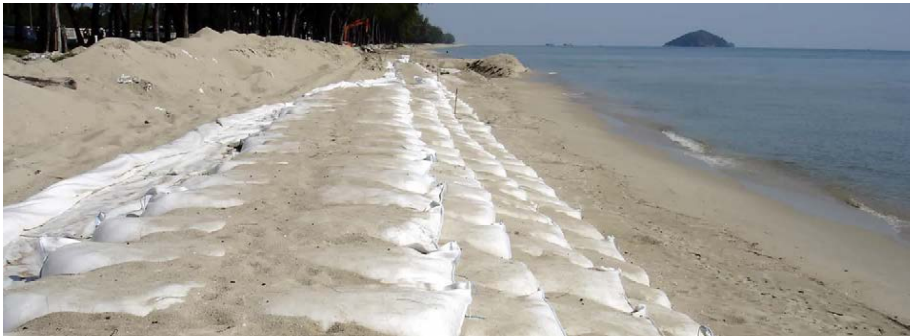
Project: coastal protection with sand containers
