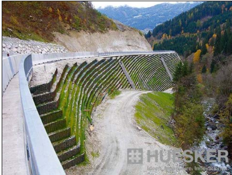
Reinforced soil walls e.g. with Fortrac®
