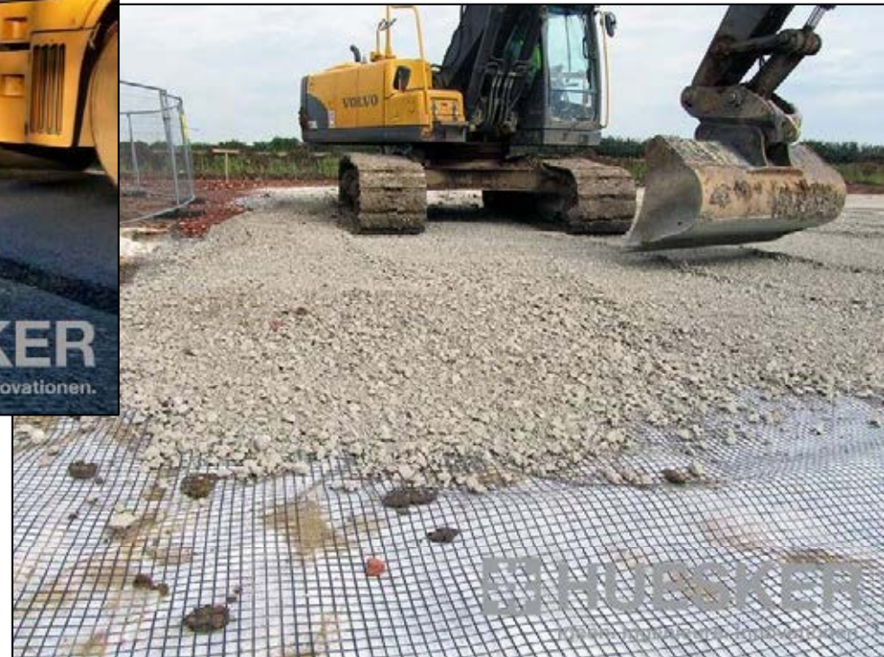
Base reinforcement
