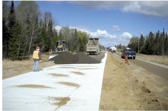
Figure 1.1.10. Rehabilitation of road Ontario Canada (copyright ROUGH project participants).
