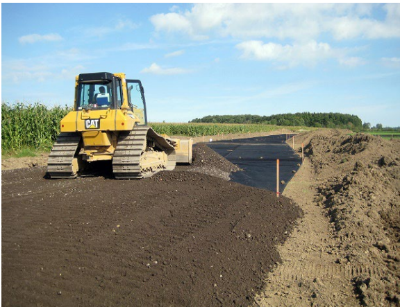
Figure 1.1.23. Construction of base reinforcement (copyright ROUGH project participants).
