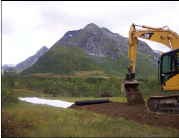
Figure 1.1.21. Embankment on soft subsoil (copyright ROUGH project participants).
