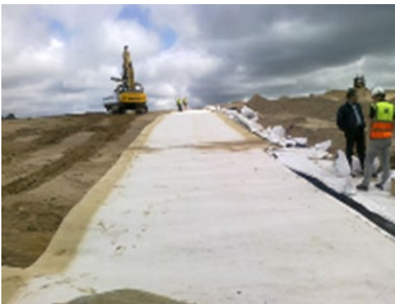
Figure 1.1.25. Solid waste disposal (copyright ROUGH project participants).
