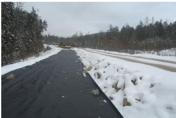
Figure 1.1.7. Construction of road in Ukraine (copyright ROUGH project participants).
