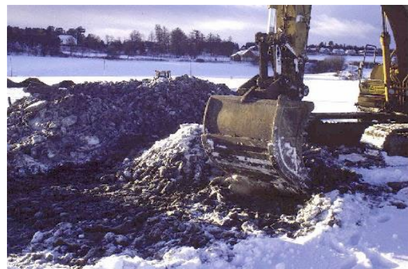
Figure 1.1.2. Winter construction works in Nordic countries (copyright ROUGH project participants)
