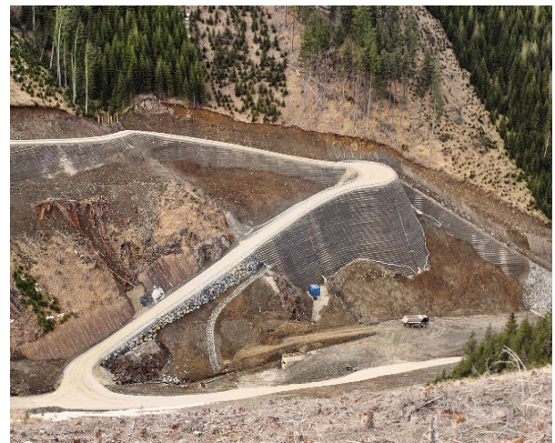
Figure 1.1.20. Reinforced soil structure (copyright ROUGH project participants).
