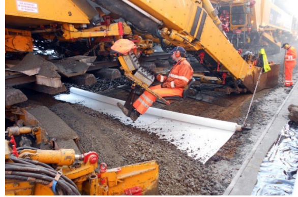
Figure 1.1.14. Base Reinforcement, construction of track beds (copyright ROUGH project participants).
