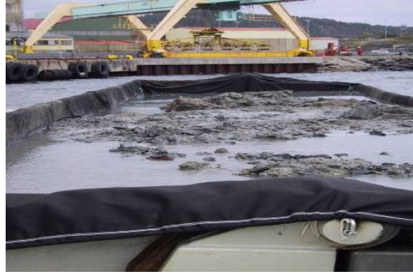
Figure 1.1.4. Geosynthetic filter in a split-bottom barge (copyright ROUGH project participants)
