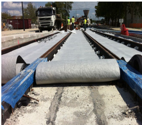
Figure 1.1.17. Drainage under a tram construction (copyright ROUGH project participants).
