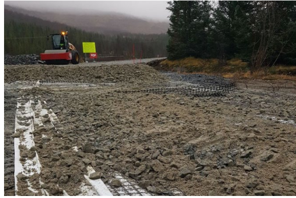
Figure 1.1.12. Road construction in Norway (copyright ROUGH project participants).
