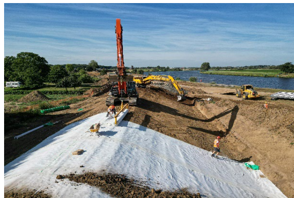
Figure 1.1.28. Construction of a dam (copyright ROUGH project participants).
