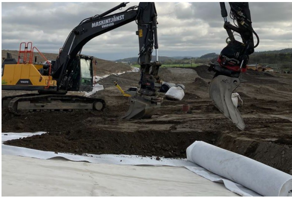
Figure 1.1.11. Construction in Lassabacka Sweden (copyright ROUGH project participants).
