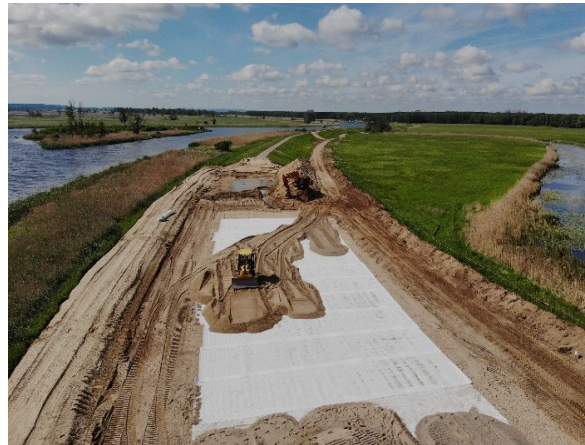
Figure 1.1.22. Embankment on soft subsoil (copyright ROUGH project participants).
