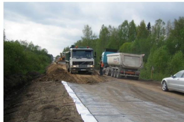
Figure 1.1.8. Construction of road in Estonia (copyright ROUGH project participants).
