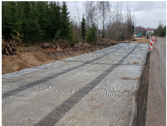
Figure 1.1.24. Construction of base reinforcement in Lithuania (copyright ROUGH project participants).
