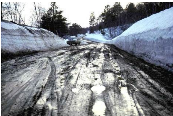
Figure 1.1.1. Gravel road during thaw period (copyright ROUGH project participants)
