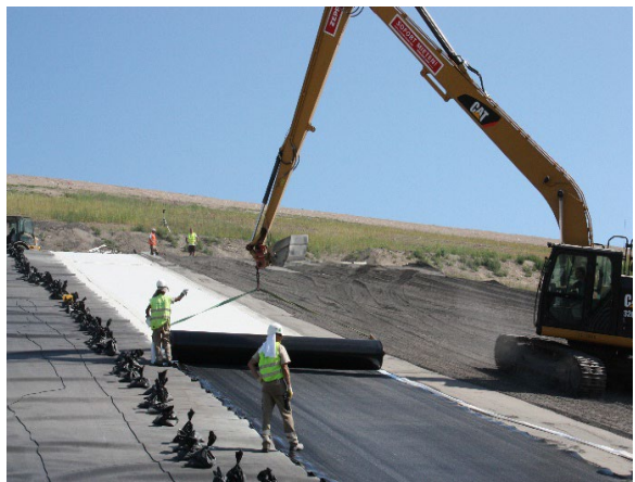
Figure 1.1.26. Solid waste disposal (copyright ROUGH project participants).
