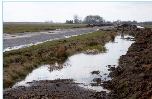
Figure 1.1.6. Challenging Ground Conditions, Soft Soil 02 (copyright ROUGH project participants)
