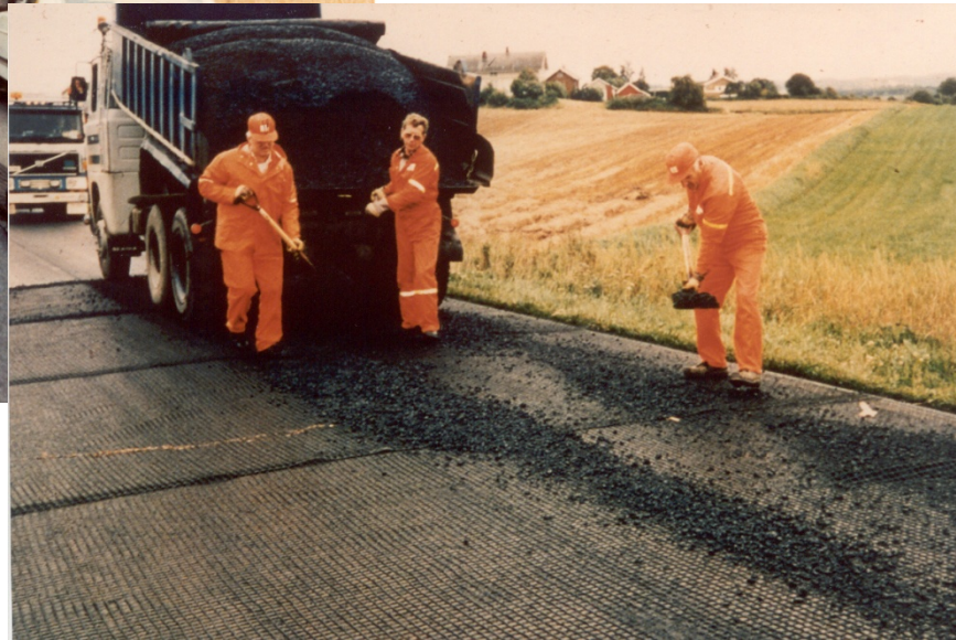
Installation and traffic on reinforcement
