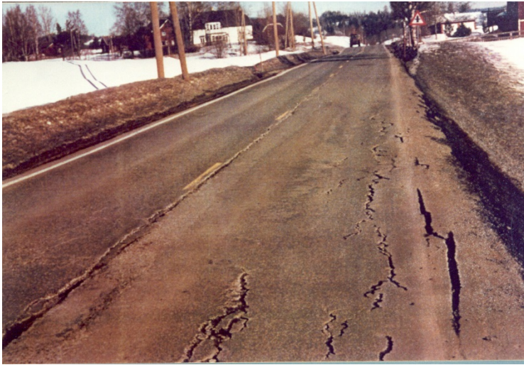
Cracking from rutting
