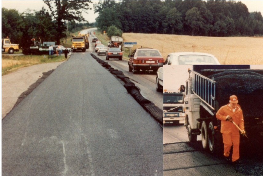
Wrinkles and overlap of reinforcement
